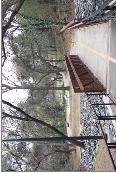
Description: Prefabricated Steel Bridge with Concrete Deck Example
